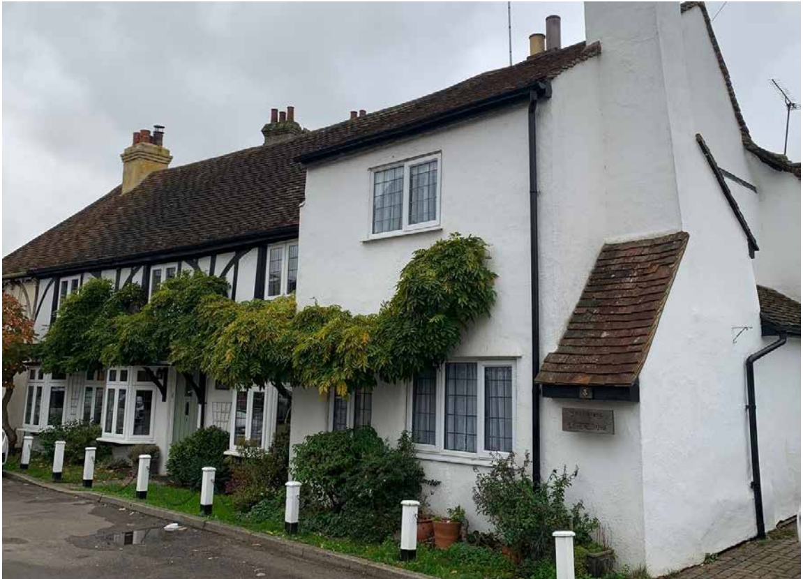
Figure 9: Tiled roof dominates in conservation area
