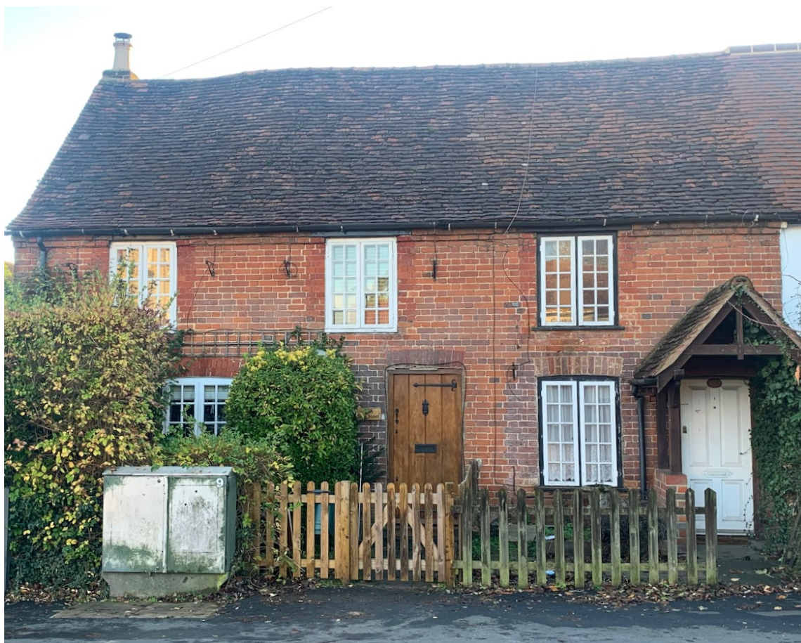
Figure 6: Timber framing of 106 & 108 High Street, encased in brick in C18th
