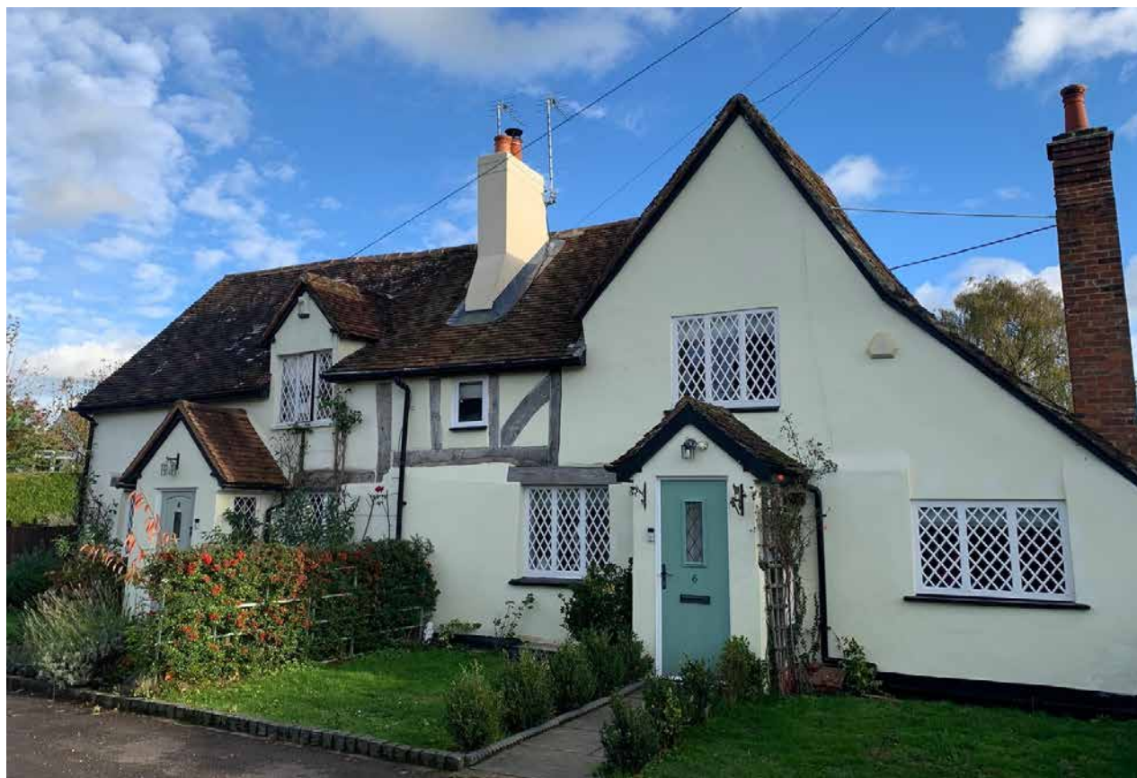
Figure 10: Bull Cottages incorporating medieval cruck and box framing
